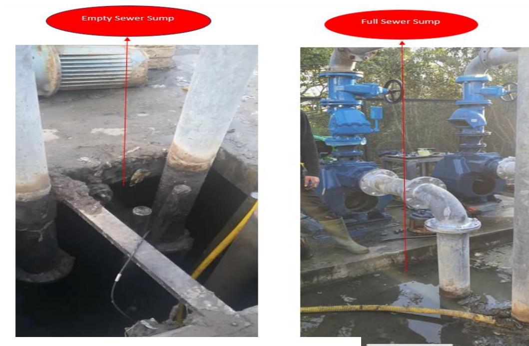
Figure 3.3 Sewer Pump station
