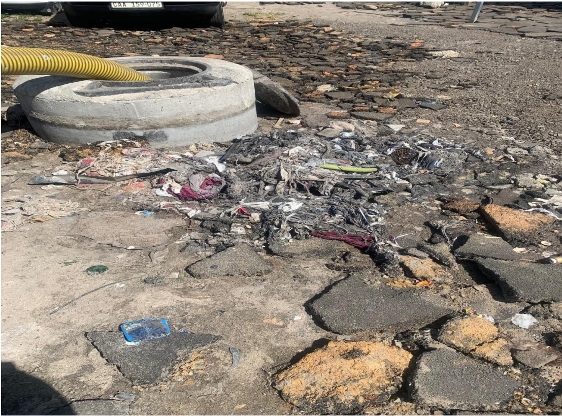
Figure 4.24: Foreign objects removed from sewers in Nyanga
