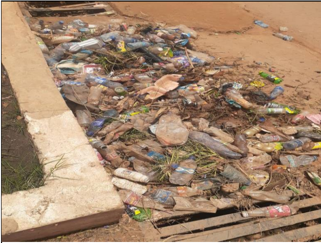
Waste disposed on top of a water channel
