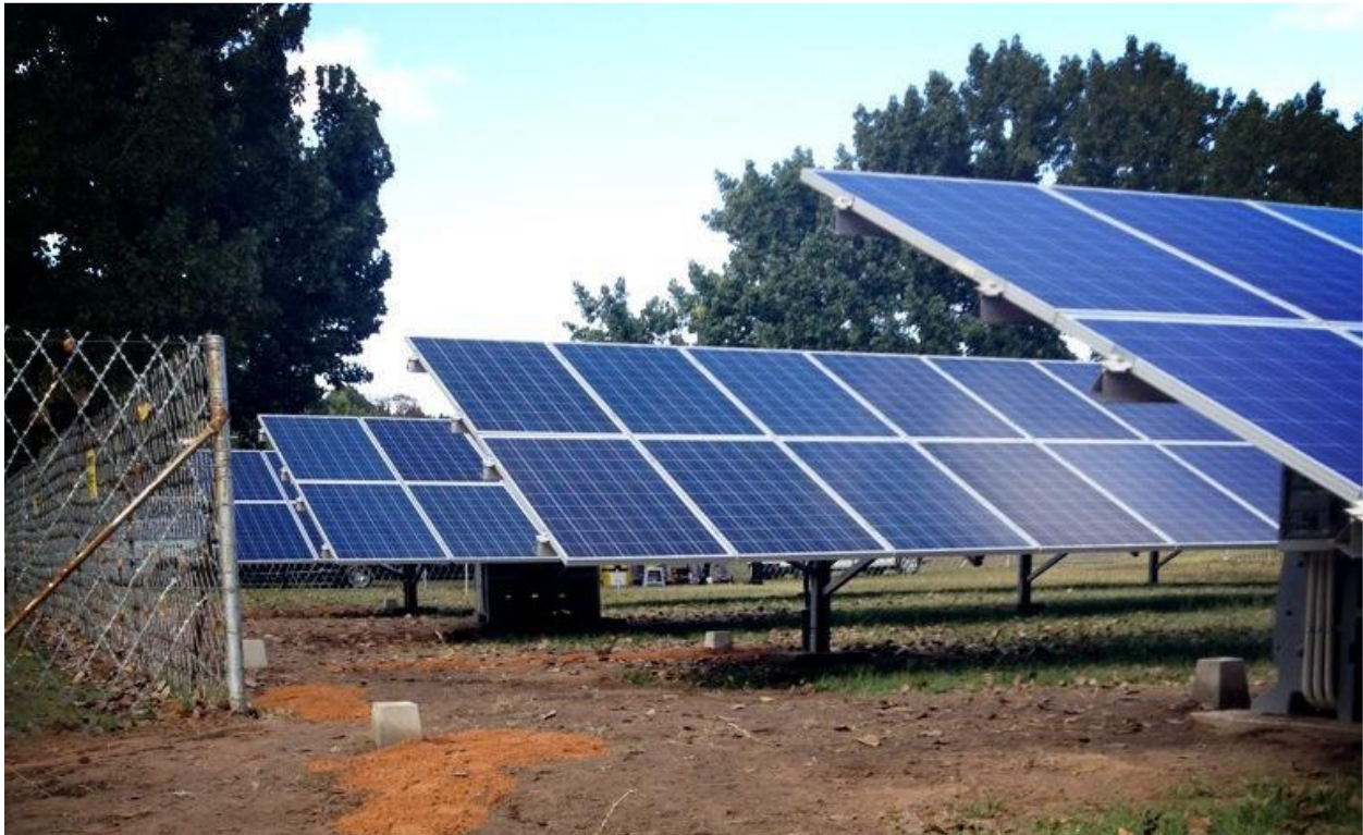
Figure 2.5: Photograph of a photovoltaic solar energy facility (tracking technology - from Sunworx Photovoltaic Systems website) (Source: Savannah Environmental (Pty) Ltd., 2013).
