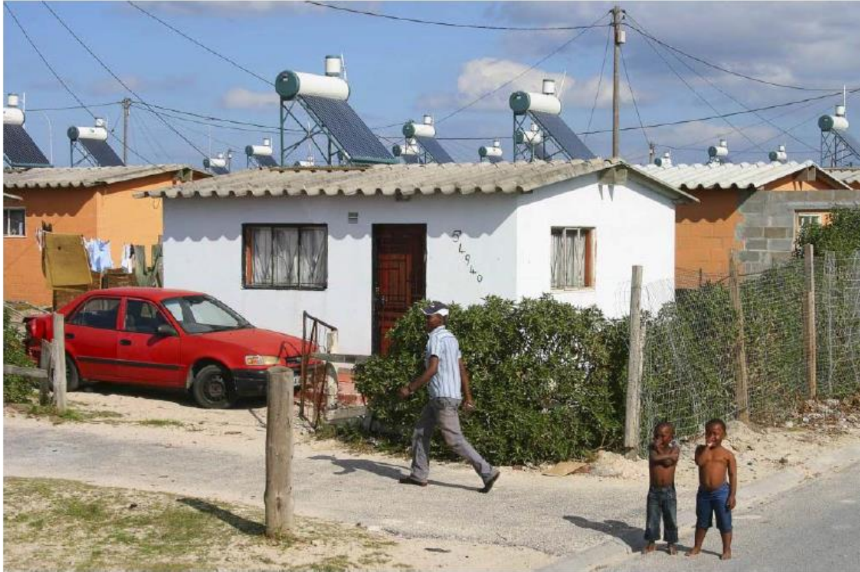
Figure 2.7: Solar water heaters installed in Khayelitsha Village, Western Cape (Source: Preston, 2009)
