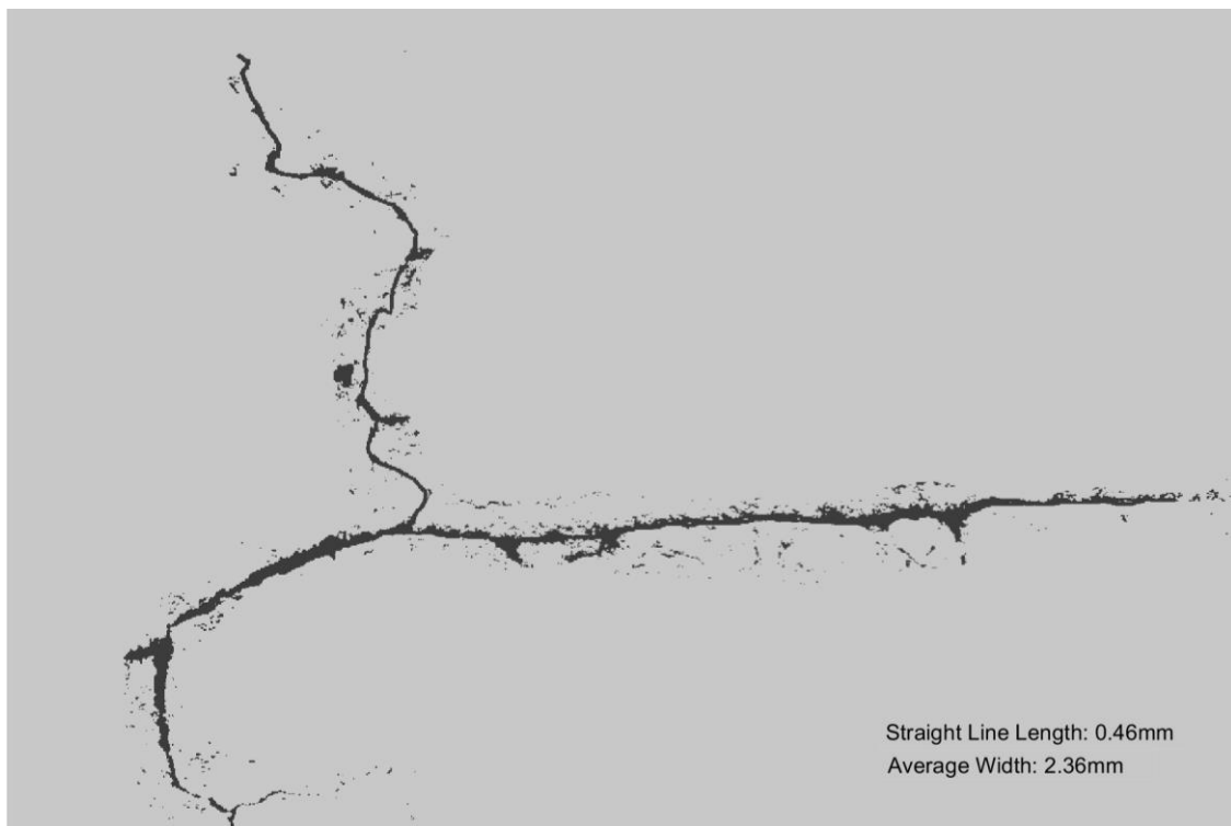
Figure C.6 Linear crack length and average crack width obtained for crack "f".
