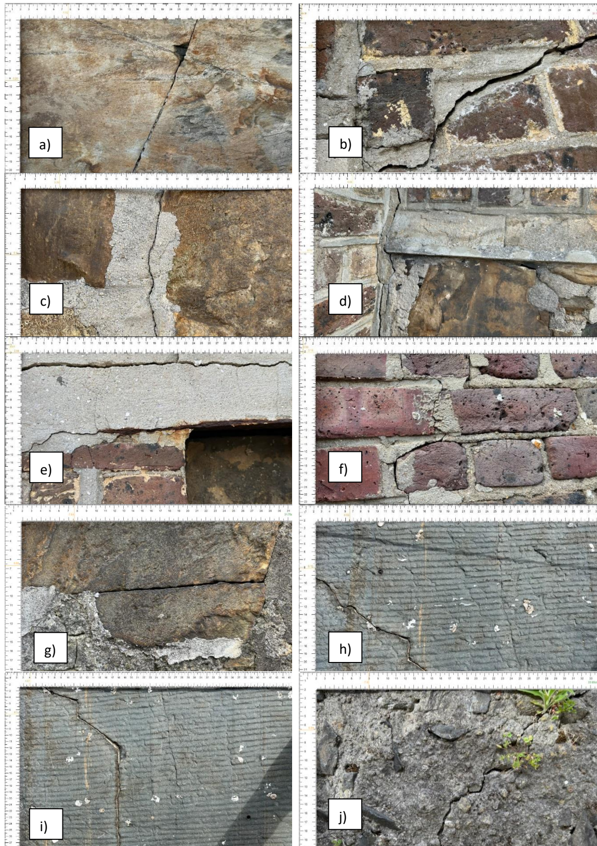
Figure 4.42 Sample of images (a) to (j) used to determine the extent of damage using image processing.
