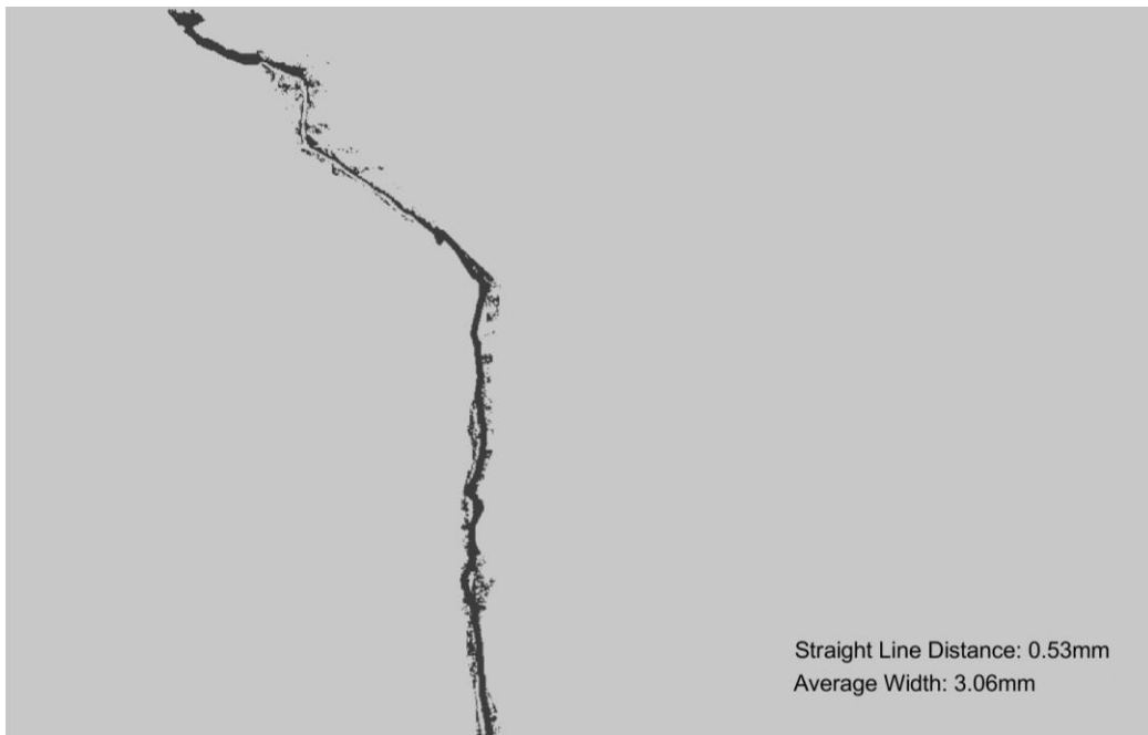
Figure C.9 Linear crack length and average crack width obtained for crack "i".
