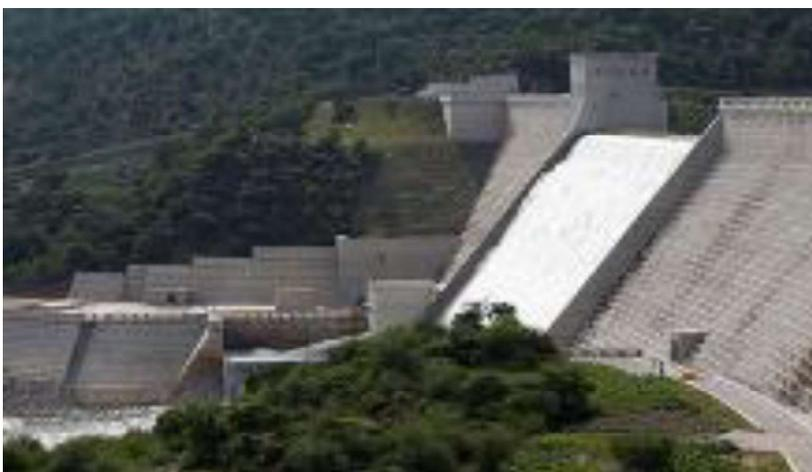
Figure 2.4 De Hoop Dam is a RCC gravity dam on the Steelpoort River, Limpopo (DWS, 2020)
