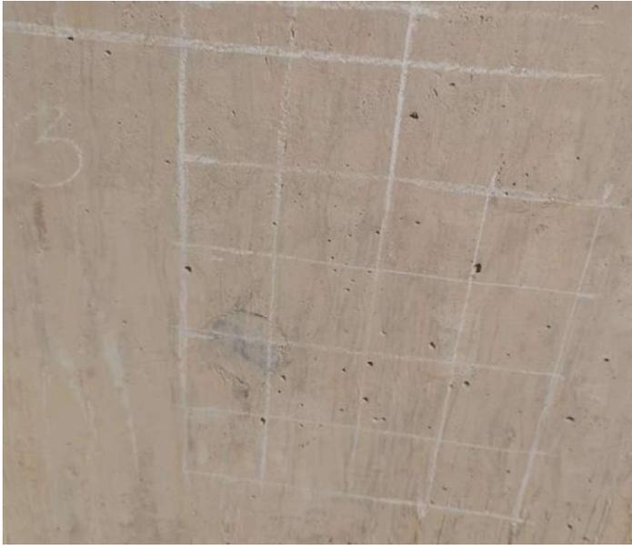
Figure 3.18 RH test square marked out on dam wall
