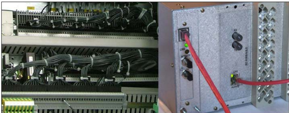
Figure 9: Comparison between hardwired communication cables and an Ethernet-based cable (Sichwart, 2012)
