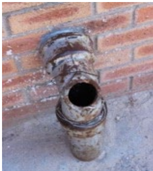
Figure 4. 36: Open sewerage outlet piping
