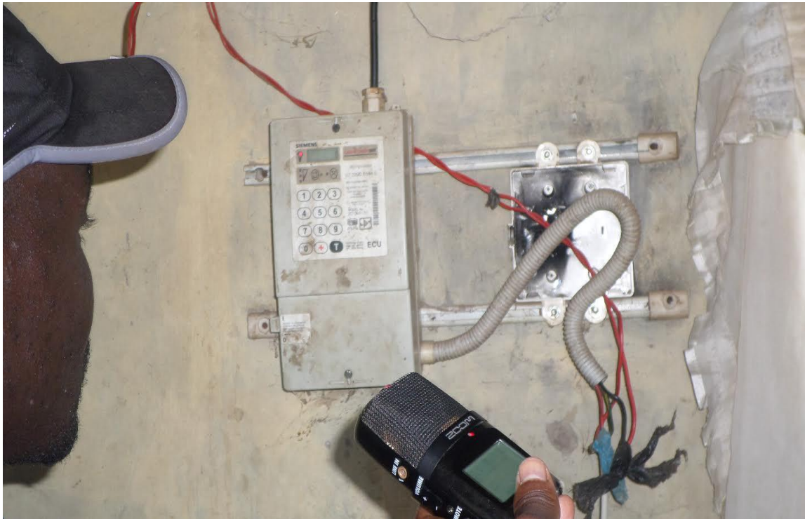
Figure 1.5: Bypassing the electricity meter (MyBroadband, 2015)
