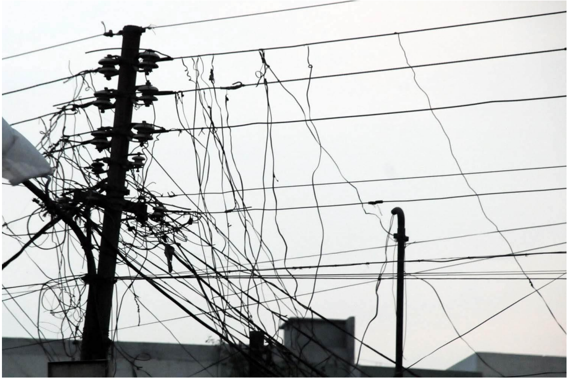
Figure 1.4: Stealing electricity directly from the distribution lines via throw-ups
