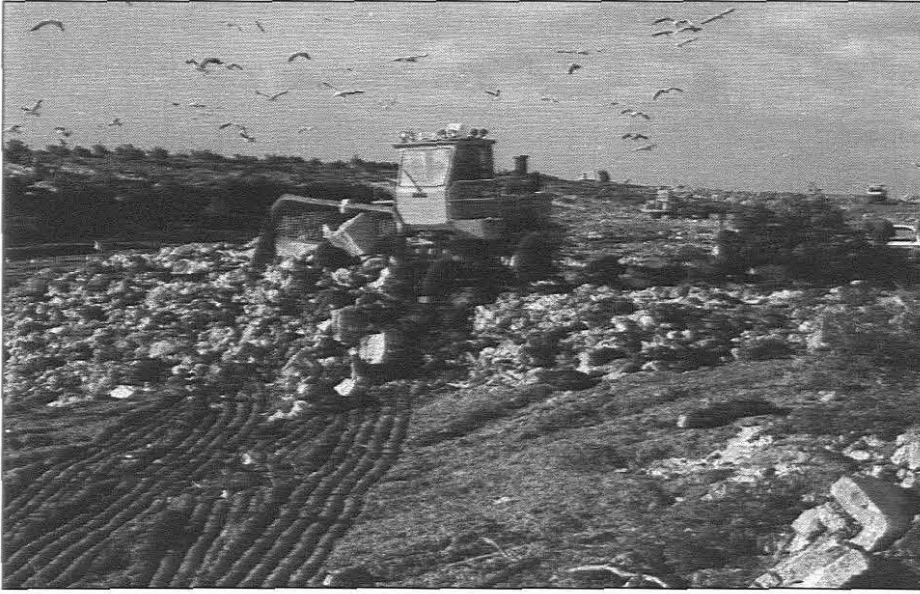
Figure (2.4): Daily covering and compacting of waste at the landfill site.
