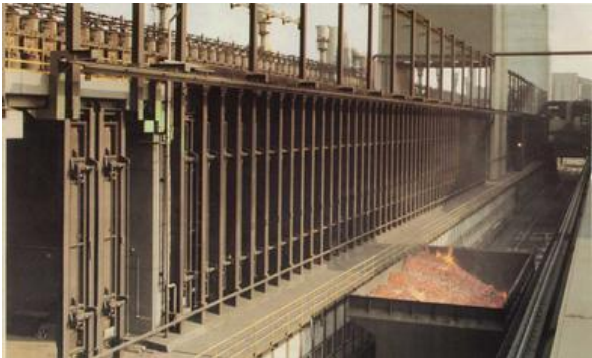
Figure 1.3 Coke side of a coke oven battery. The oven has just been "pushed" and railroad car is full of incandescent coke that will now be taken to the "quench station".
