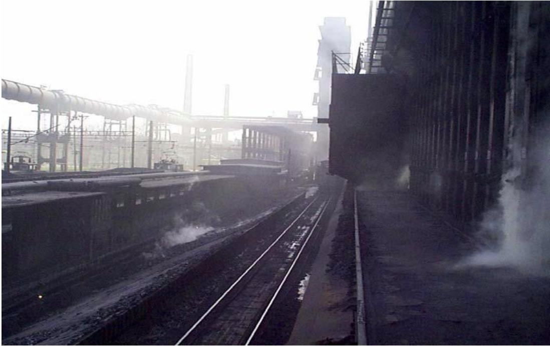
Figure 1.6 Coke oven back side work environment
