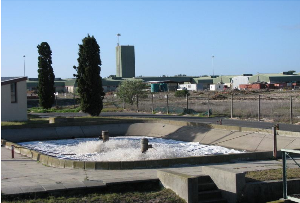
Figure 4.42: MRC Sewage Treatment Works (STWs)
