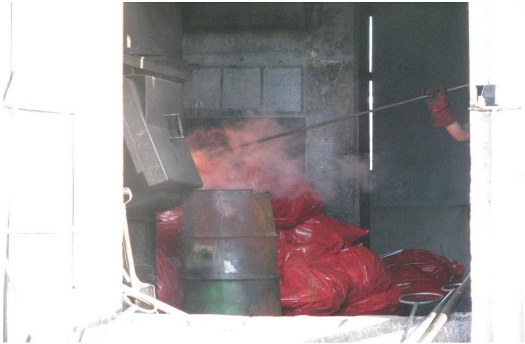
Figure 4.34: Hot bottom ash removed manually and escaping to the atmosphere
