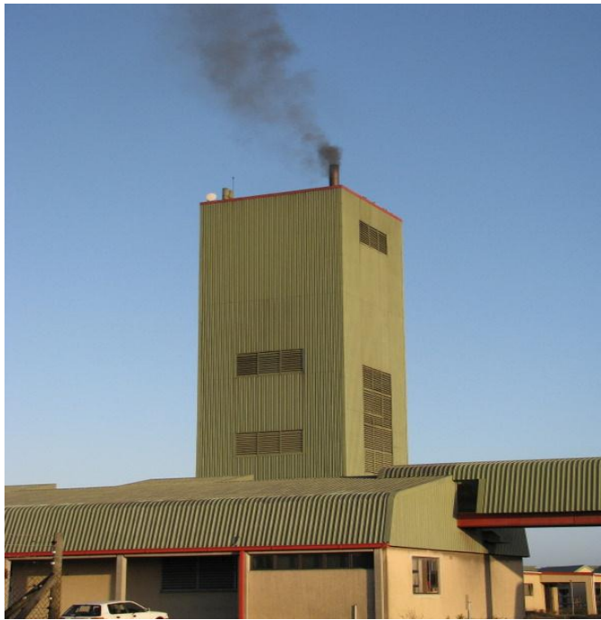
Figure 4.31b: BCL MWM incinerator emitting black smoke
