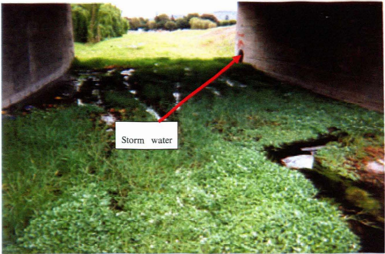
Plate 3: Storm water drain under the bridge at Amandel Road
