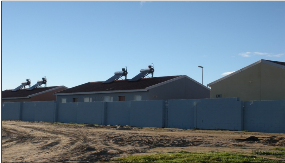
Figure 5.19: Some houses have been completed and occupied.
