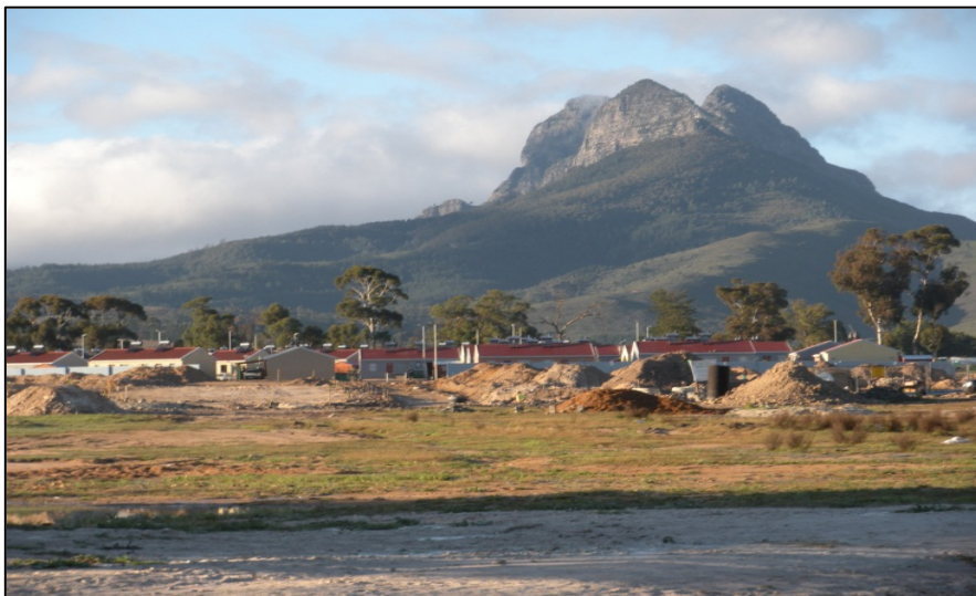
Figure 5.18: Construction activities has commenced on the site.
