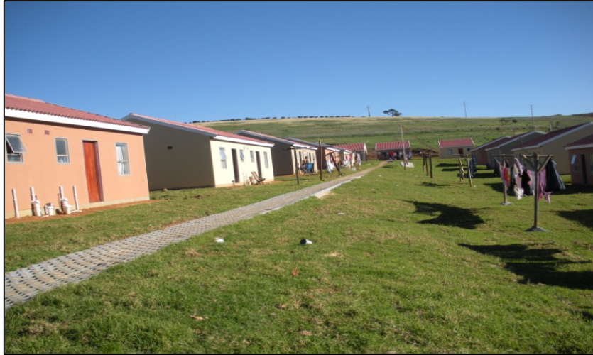
Figure 5.11: Many of the new completed houses have been occupied by residents.
