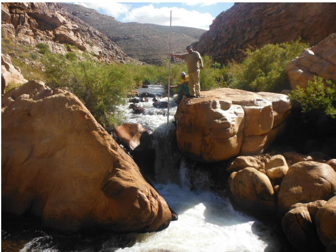
Figure 3.32 Black bass barrier in the Matjies River. The barrier is a single fall with a drop of 0.97 m.
