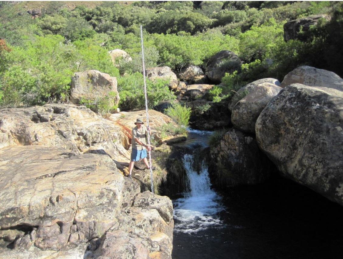
Figure 3.22 Black bass barrier in the Jan Dissels River. The single fall barrier has a drop of 1.17 m and is located in the Cederberg Wilderness Area.
