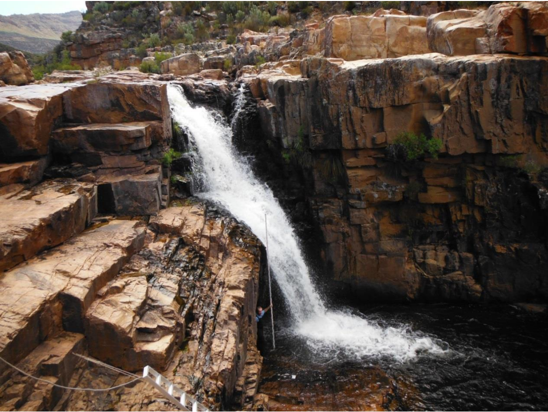
Figure 3.36 Black bass barrier in the Twee River. The total height is 7.35 m and the effective drop is the bottom fall that is 3.5 m high.
