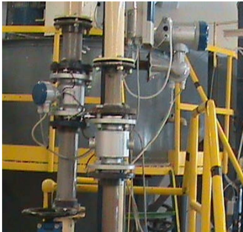
**Figure 3.6: Magnetic flow meters**
