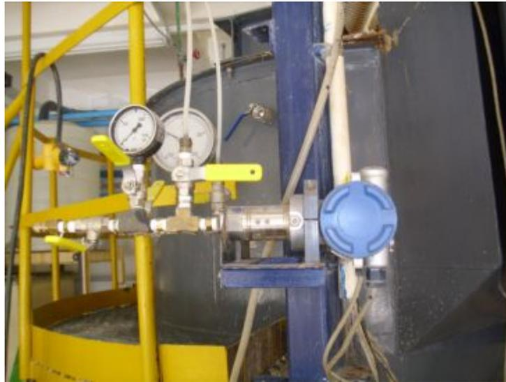
Figure 3.4: Point Pressure Transducer (PPT)
