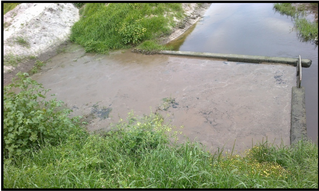
Figure 2.5: Sludge from the secondary treatment (MPWWTP, 2012)
