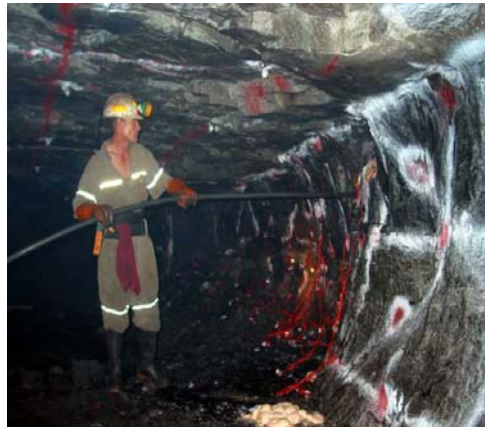
Figure 1.2: Application of explosive emulsions underground ( )
