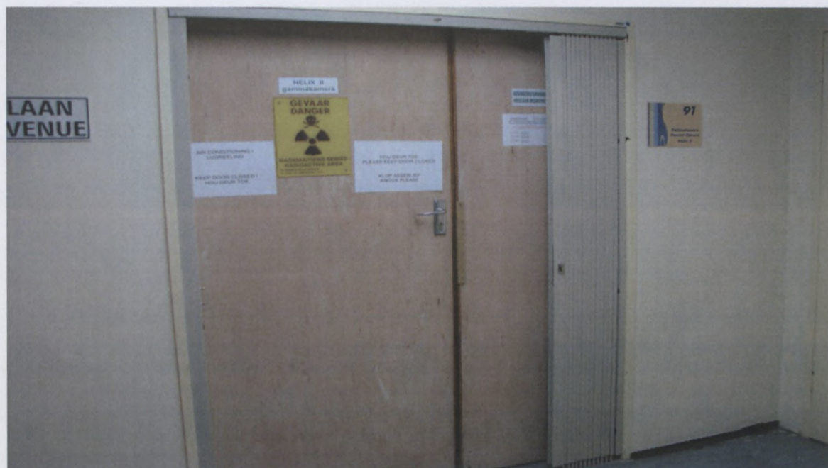
Figure 4.9: Radioactive waste storeroom without proper signage
