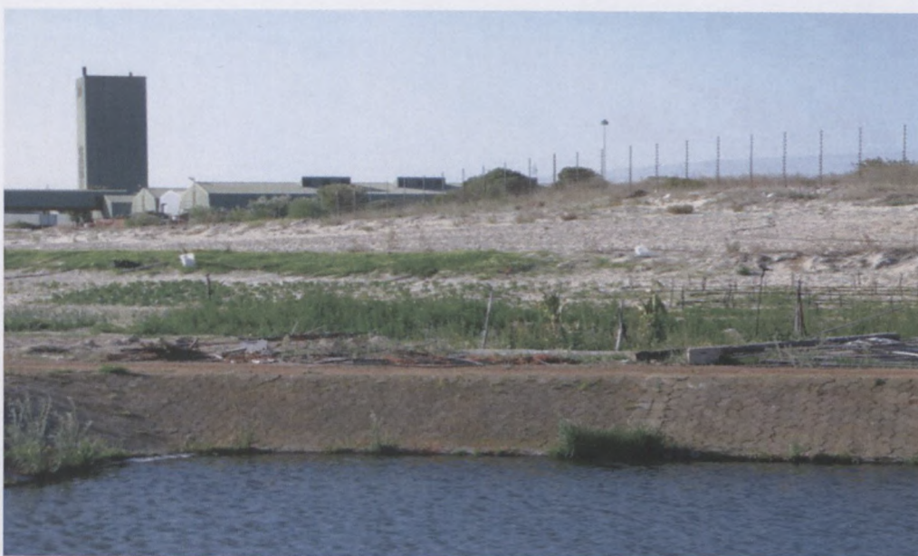
Figure 4.43: Final effluent retention pond of the MRC STWs
