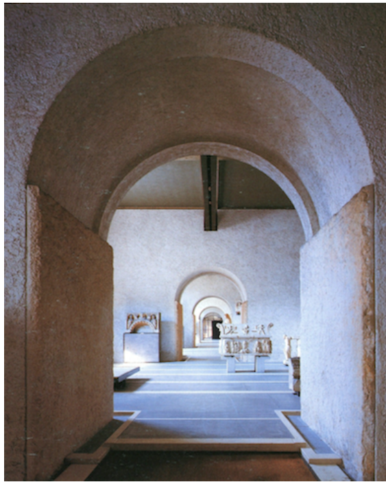
Figure 5.26 Detached inserted floor
