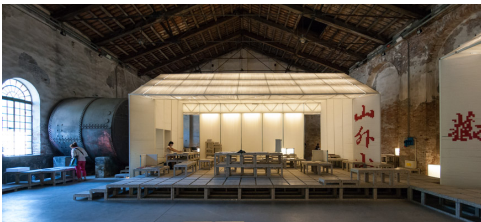
Figure 5.25 Raised detached floor
