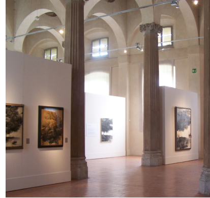
Figure 5.29 Disconnected detached wall
