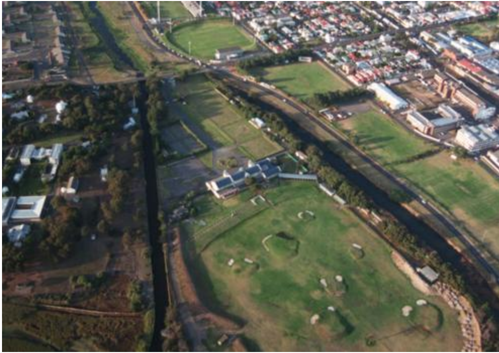
Figure 4.8: An aerial view of The River Club. File picture: Andrew Ingram (SRK Consulting (South Africa) Pty Ltd, 2016)
