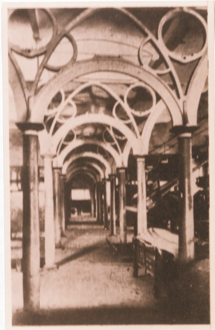
Figure 2a. Interior view of the Stanley Mill, Gloucestershire, built in 1813. Note the circular bearing shells which carried the gaint turning shafts carrying mechanical power to the machinery. ( Source : MacMillan 1979 ).
