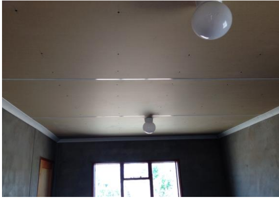
Fig. 24 Represent a complete ceiling installed with electric lights installed.
