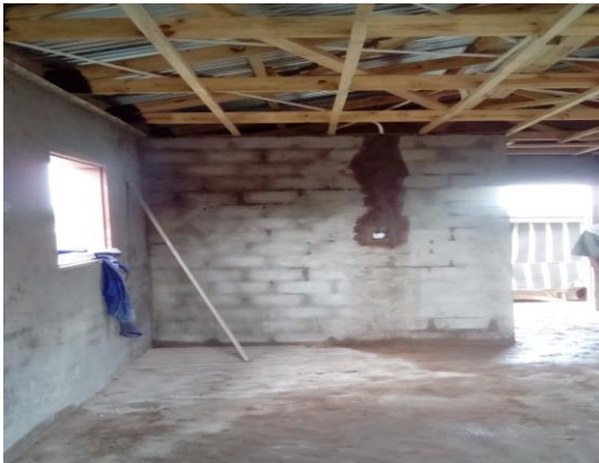
Fig. 18 Represent the brandering installed at 500mm c/c and electric conduit pipes.
