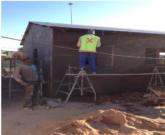
Fig. 25 Represent plastering works in progress.
