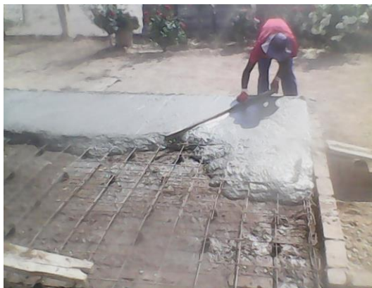
Fig. 7 Represent the casting of concrete floor slab.
