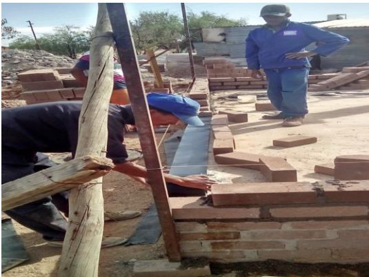
Fig. 10 Represent the laying of dpc for superstructure.
