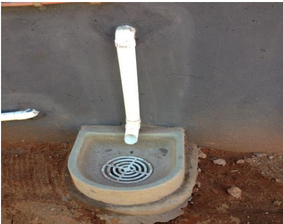
Fig. 29 Represent the gully stone installed correctly.
