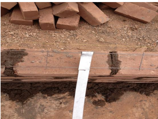
Fig. 11 Represent the hoop-iron tied to the brick-force in every fourth course.
