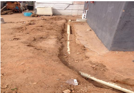
Fig. 30 Represent waist pipe installed ready to be back-filled.
