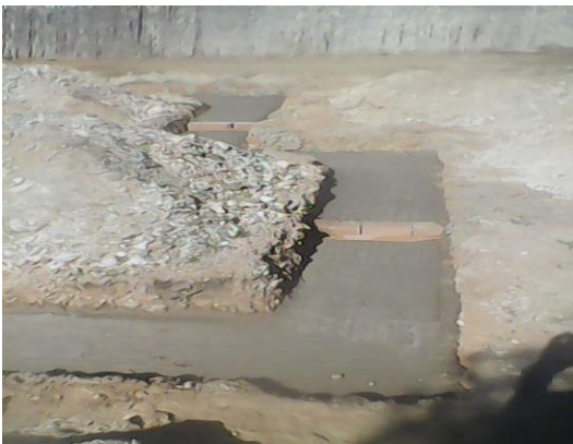
Fig. 3 Represent a step footing.
