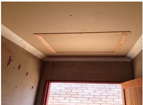
Fig. 23 Represent a complete ceiling, cornice with trap-door.
