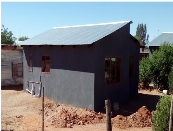
Fig. 31 Represent a complete house (roof, window panes, plumbing and paint).
