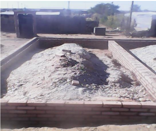
Fig. 5 Represent a complete foundation brickwork.
