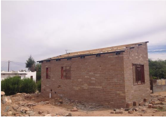
Fig. 16 Represent a complete and correct positioned roof trusses.
