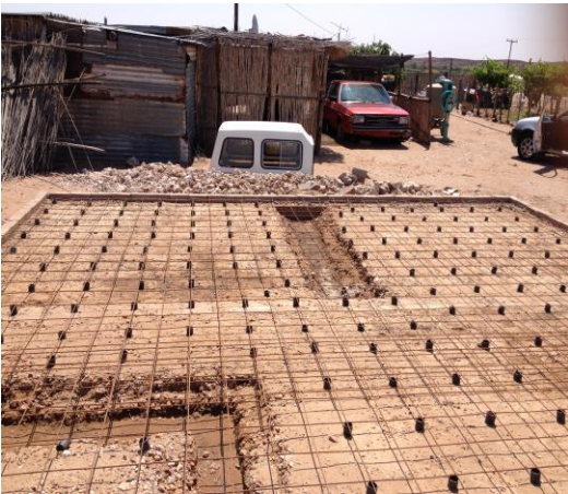
Fig. 6 Represent a backfilled, stumped, leveled with spacers and mesh wire.
