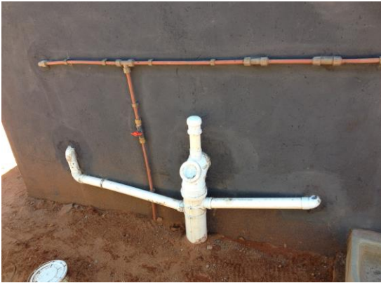
Fig. 28 Represent a complete Plumbing works (water and sewer pipes).
