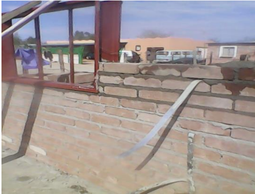
Fig. 13 Represent the window frame installed.
