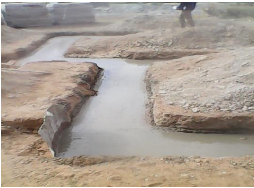
Fig. 2 Represent 600mm x 250mm footing (high strength 25Mpa).
