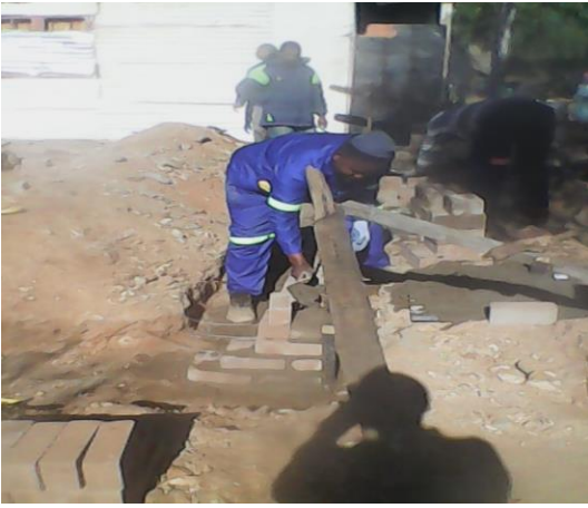
Fig. 4 Represent a two skin foundation brick-wall.
