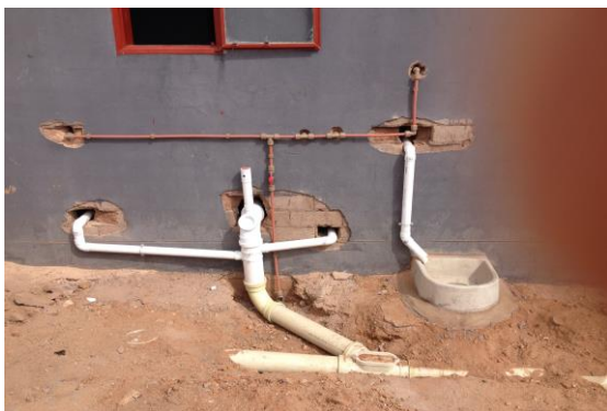
Fig. 27 Represent plumbing works in progress (sewer and water pipes).
