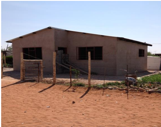
Fig. 26 Represent a house with complete plastering and roofing.
