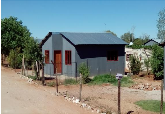
Fig. 32 Represent a complete house with door installed.
