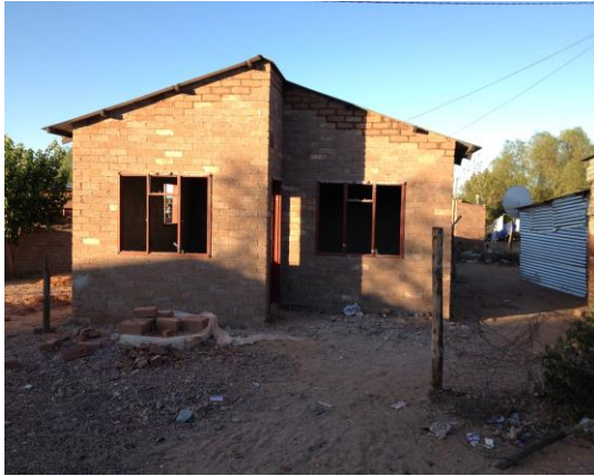
Fig. 17 Represent a complete roofing with beam filling.
