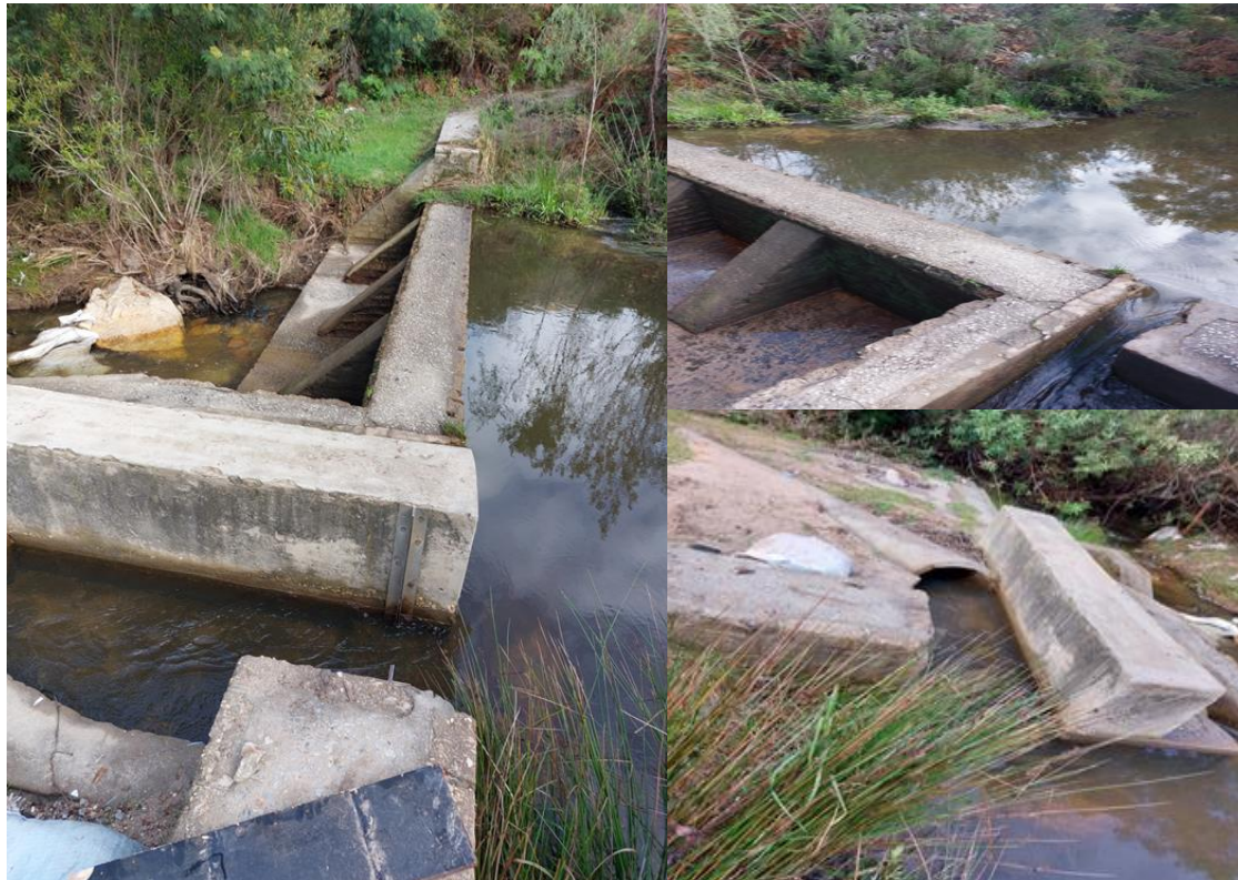
Figure 4.7: The weir in the Platkloofrivier which is used to obtain irrigation water
