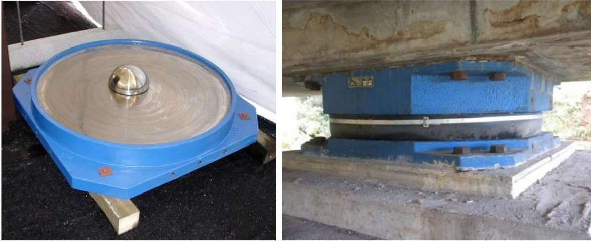
Figure 2.3: Cross section of friction pendulum system (FPS), open and installed (Adapted from Robertson (2010))
