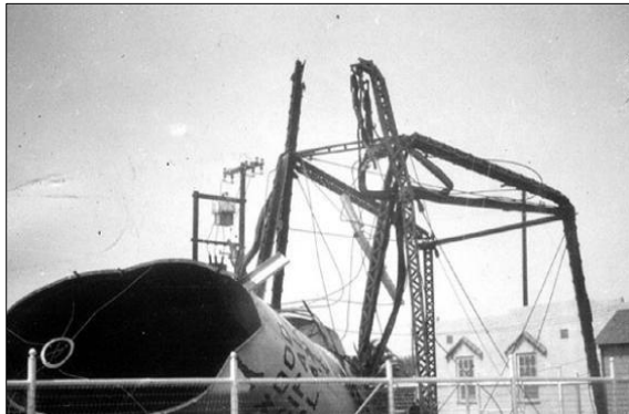
Figure 1.1: Support frame collapse of elevated steel water reservoir, 1933, Long Beach (Adapted from NZSEE, 2009)
