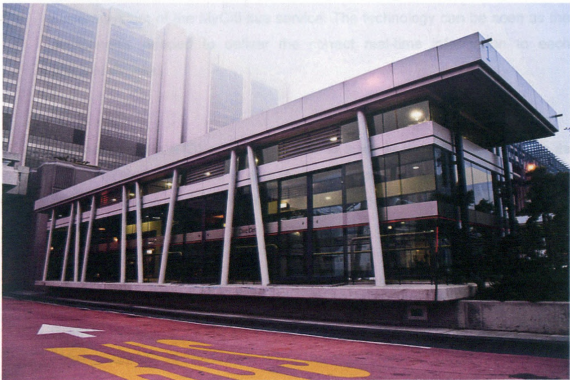
Figure 8.10: Main station at the Civic Centre
