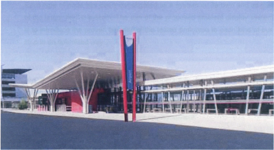
Figure 8.9: Main station at Airport
