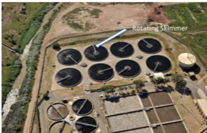
Figure 2.1: Circular clarifier with visible surface skimmer. Courtesy CoCT Wastewater treatment works.
