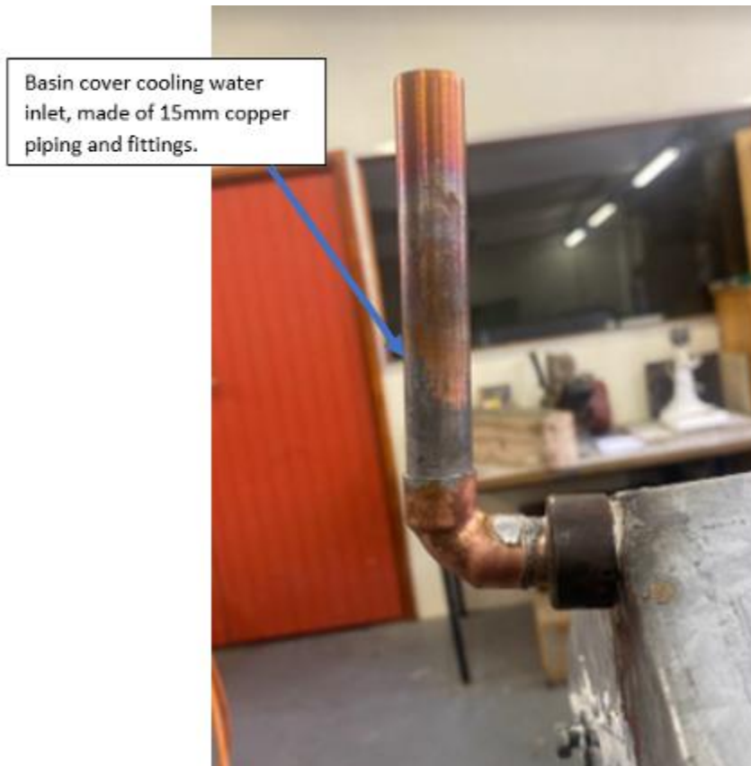
Figure 3.7: Cooling water inlet
