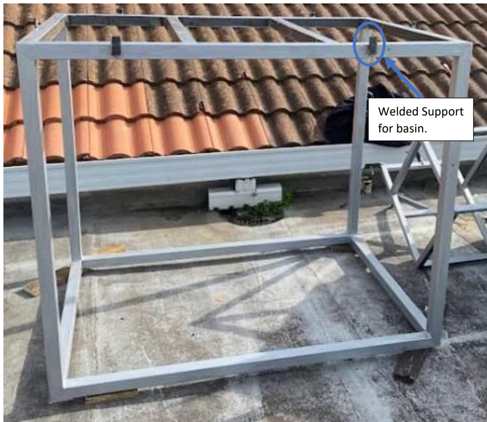
Figure 3.14: Water basin frame
