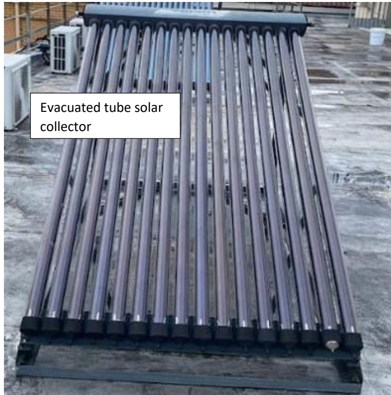
Figure 3.25: Evacuated 16-tube solar collector
