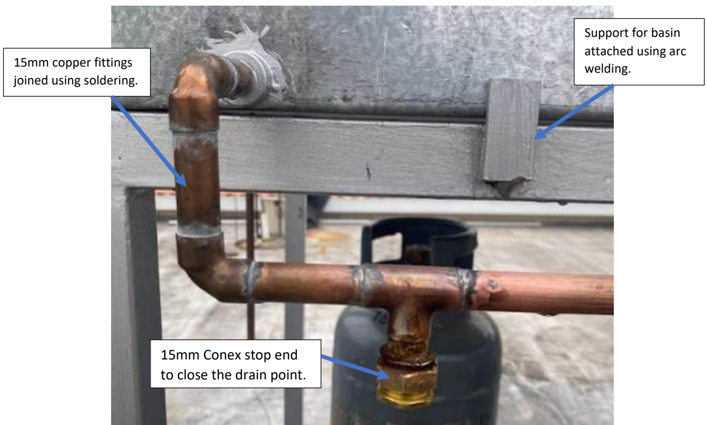
Figure 3.20: Basin to ETSC connection (drain point)
