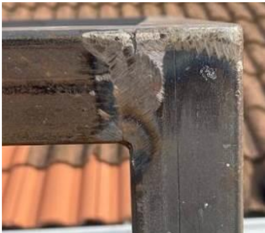
Figure 3.15: Clean arc welding joint
