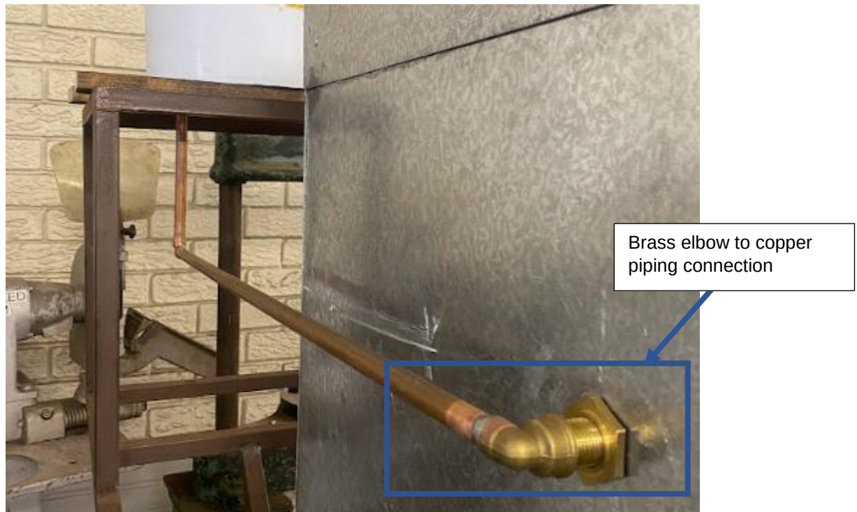
Figure 3.11: Primary tank to basin connection
