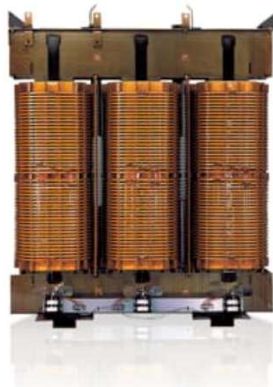
Figure 2.7: Open wound transformer (VPE) (Hitachi, 2022)
