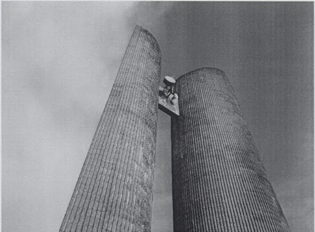
Figure 54. The twin steeples of the Kuilsrivier De Eike DRC, which in plan, repeat the two confronted semi-circles of the plan of the main church.
