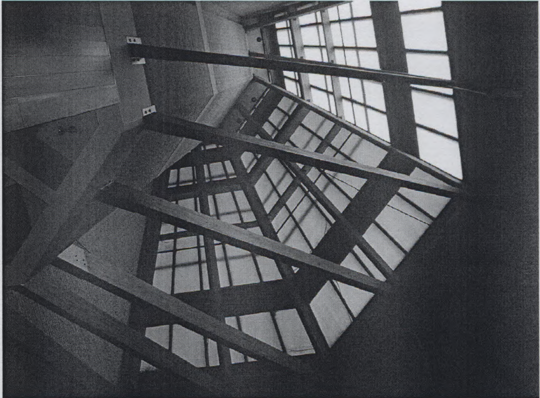
Figure 26. Interior of the Welgemoed DRC looking up the tower behind the pulpit, which casts a concealed 'heavenly' light on the pulpit. This is the only source of natural light within the auditorium.
