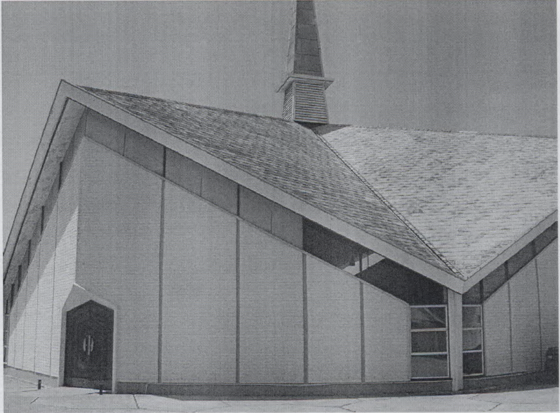
Figure 21. Exterior of the Vasco DRC.
