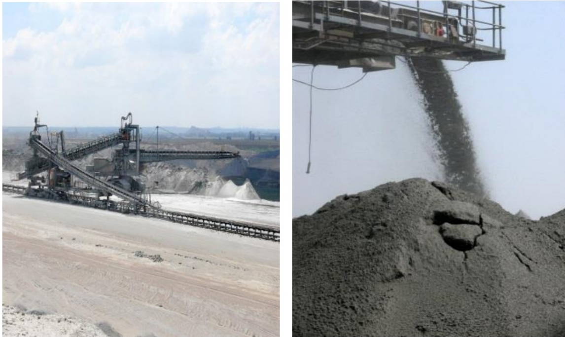
Figure 2.2: FA disposal site near one of Eskom power plant in the Mpumalanga province.
