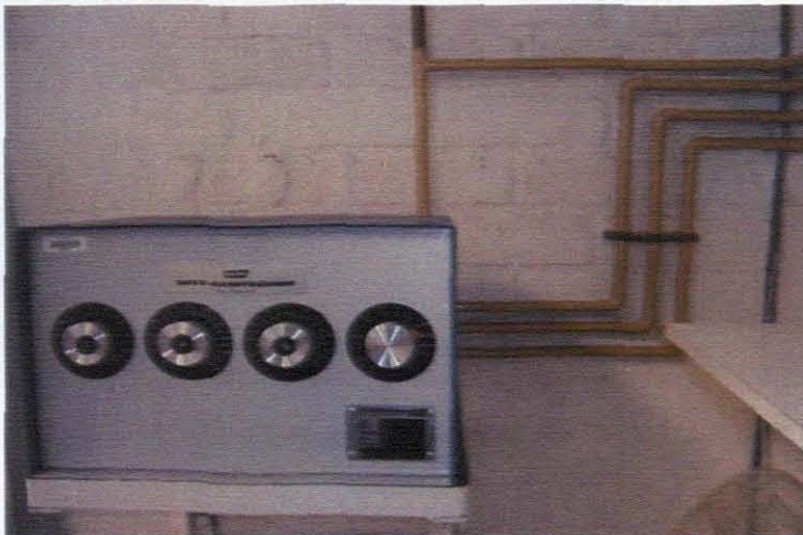
Figure 7.6: Depicts the automatic gas mixer used for the welds.
