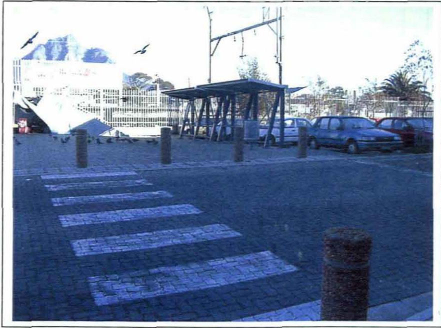
Figure 6.10 A raised pedestrian crossing and bollards define the pedestrian environment.
