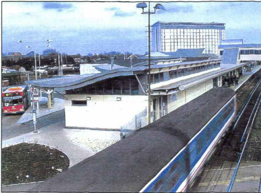
Figure 5.5 Good practice. Upgrades to this intermodal transport interchange were the result of a partnership between several public and private role players
