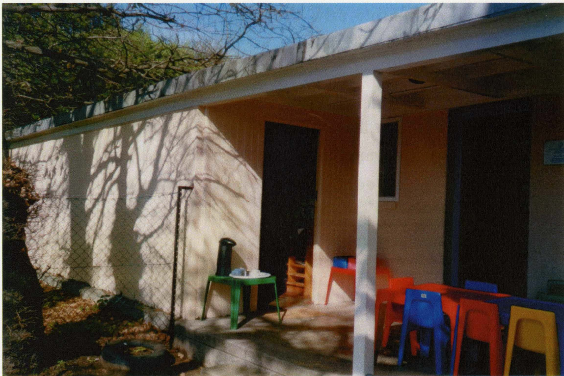
Figure 4.3 The front view of the house.
